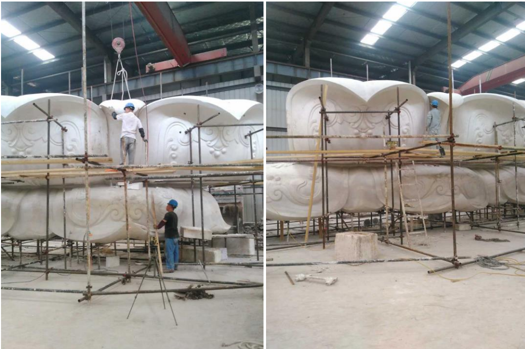
1:1 lotus foam model assembly and modification
